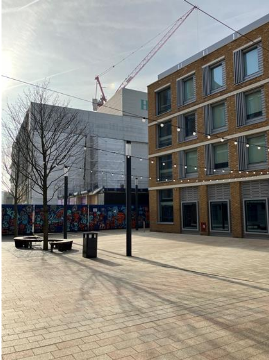
Image (left): View of partially constructed Block C podium with former Printworks building in the background.
